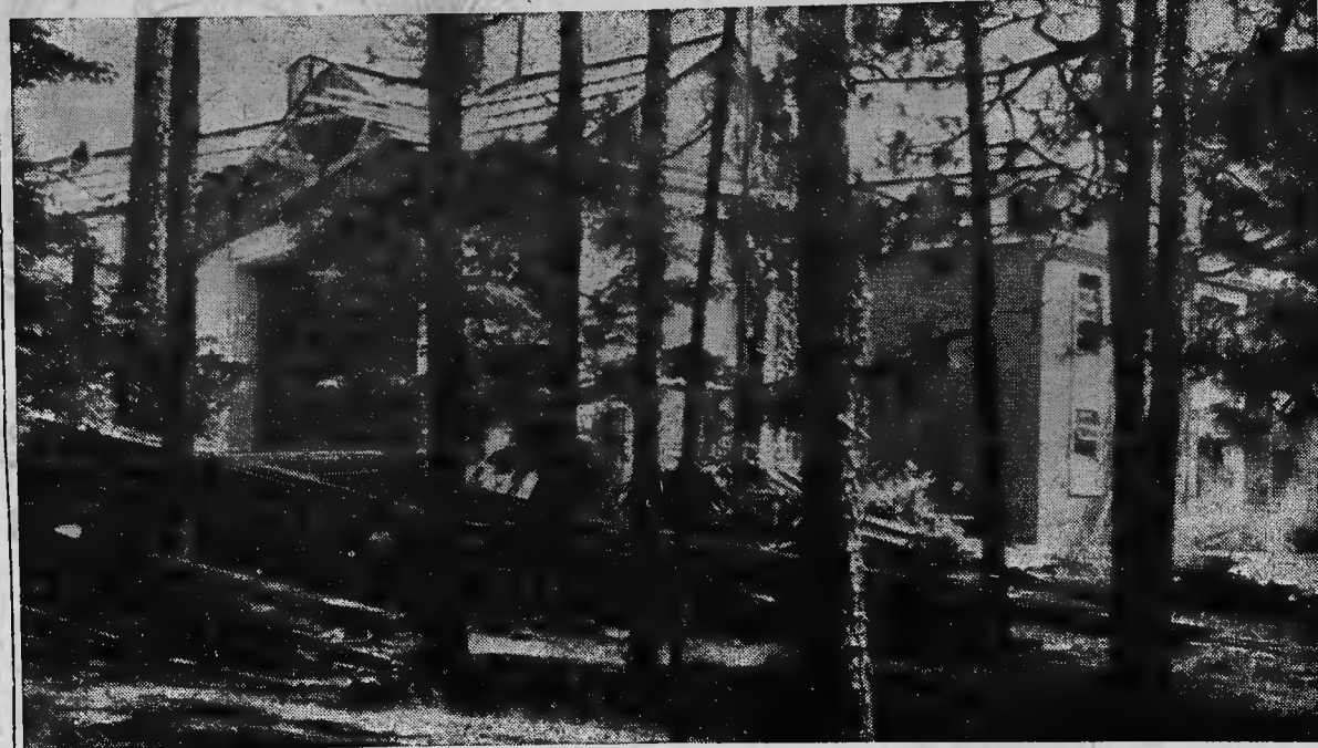
New High School Goes Up As Old Building Comes Down
