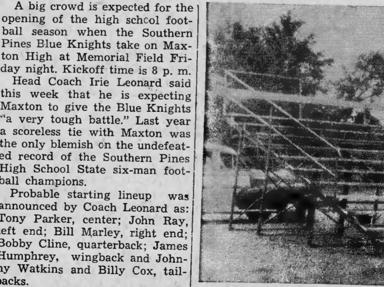
NEW BLEACHERS —These two new sets of bleachers, each accommodating 110 persons, bring the total seating capacity at Memorial Field to 550. Weather-resistant treated planks form the seats. The welded steel frames include hand rails at sides and guard rail at the back. In this photo, volunteer workers are putting finishing touches on the installation. Each set of bleachers cost $415. One was paid for from donations at summer softball games, the other from proceeds of football programs published by the Blue Knights Club, an organization of adults who are interested in high school athletics. (Pilot Photo)
