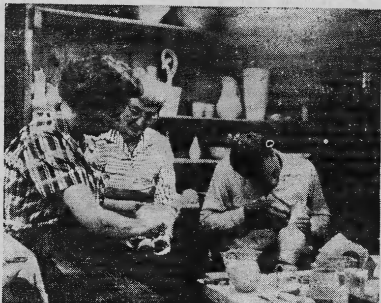
FETTLING, the process of removing blemishes on mold-formed pottery, is a job that requires the able hands of all three partners in Sandhill Ceramics, newest craft in this area. Pictured here, left to right, are Miss Mildred Gruebl, Mrs. Marion de Costa, and Don Moore, who operate the hobby turned business. (Pilot photo)
