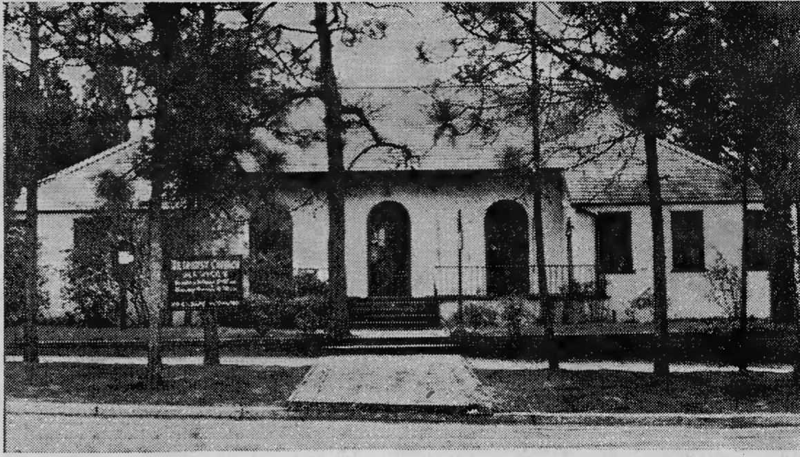
CIVIC CLUB BUILDING—This building of many uses was erected by the Southern Pines Civic Club in 1925 and is the official home of the club. Some of the various capacities in which the building has met community needs are given in the accompanying club history; one not
