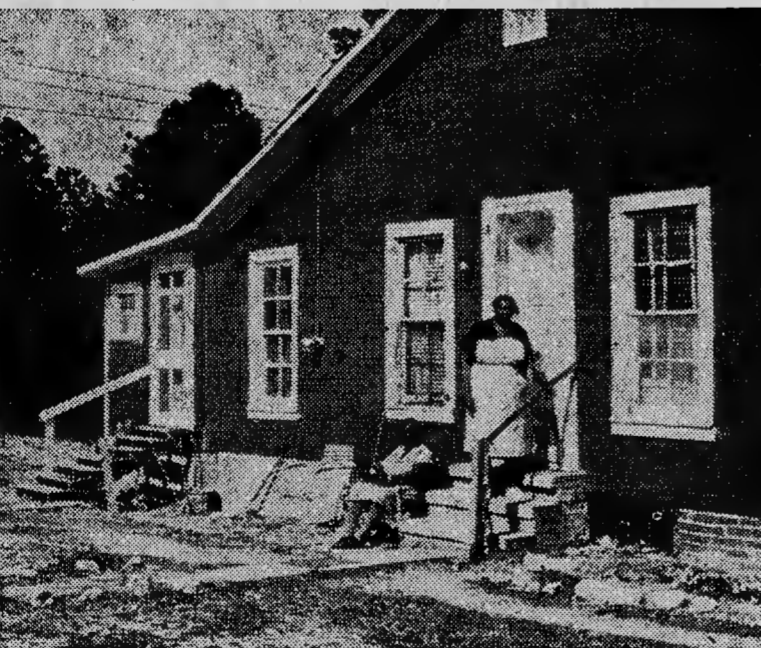
THE LEAK HOME has had quite a face-lifting, outside and in, which should add greatly to its value in the boarding home program of Moore County's Department of Public Welfare.
