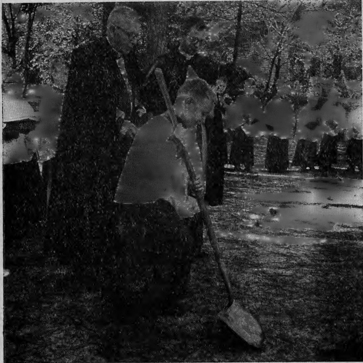
GROUND BREAKING CEREMONIES for the new children's building at Emmanuel Episcopal Church were conducted as part of the regular service Sunday morning. Young Robert Dudley, son of Mr. and Mrs. E. K. Dudley of Pinehurst, is shown here in the traditional turning of a shovelful of dirt. He followed the Rev. Martin Caldwell, rector, and the Rt. Rev. Edwin Penick, Bishop of the North Carolina Dio-
