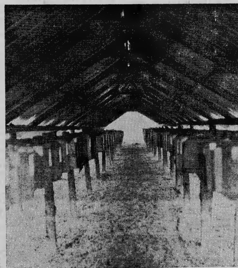
MINKS' HOME—On either side of this center walkway down the middle of this sideless shed are dozens of cages, each containing a mink, suspended above the ground, at right angles to the center walk. This view shows a "den" or box for each mink, on the inner end of each cage. The roof is of plain sheet metal over the rafters and both sides and the ends are open, allowing plenty of air circulation. This is one of two such sheds at the Pine Needles Mink Ranch. (Pilot photo)
