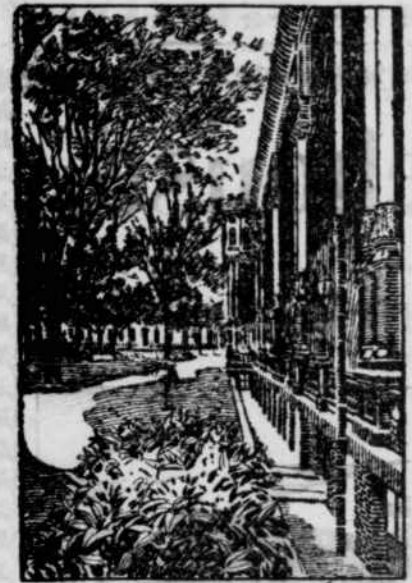
COURT OF ONE OF THE LEADING HOTELS AT SARATOGA.
