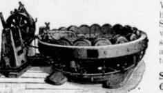
We have West's hydraulic TIRE SETTER with which we can set the tires on a wagon in fifteen minutes.
