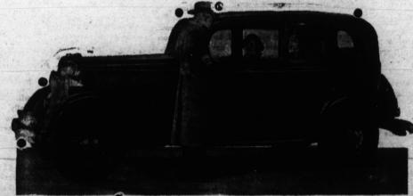
new Ford V-8 for 1934. The de luxe Tudor is shown above. Dual down draft carburstion and manifold give the engine greater power, the car increased pickup and speed. A clear-vision body system also is introduced in the new Fords.
