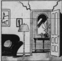
**CRACKED WALLS**—Often caused by uneven settling of footings and foundation. Skimping on footings in either size or concrete mix is poor economy.
