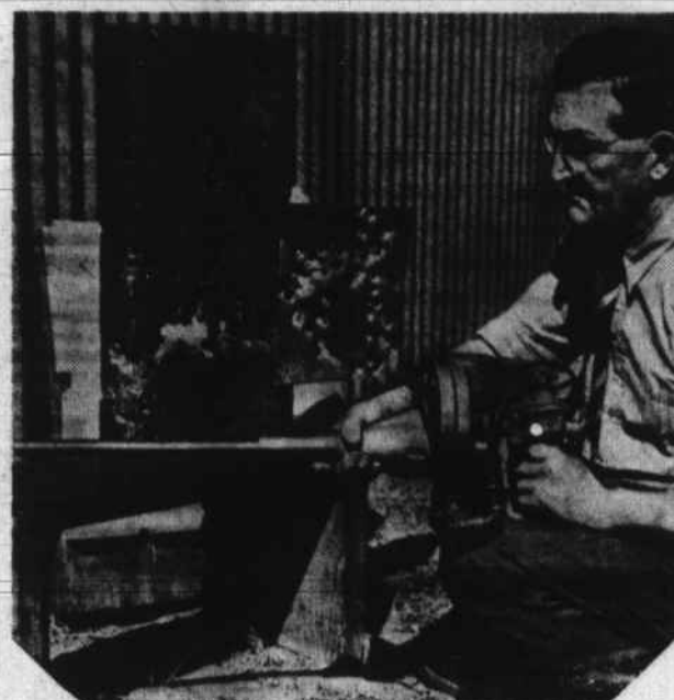
W. B. Hale, co-inventor, demonstrates the power of his new mystery machine gun in tests at Los Angeles. Shown with the gun, which is reported to fire 10,000 shots a minute, are the oak planking and armor plate that were perforated by the steel ball bullets. The gun operates on compressed air.
