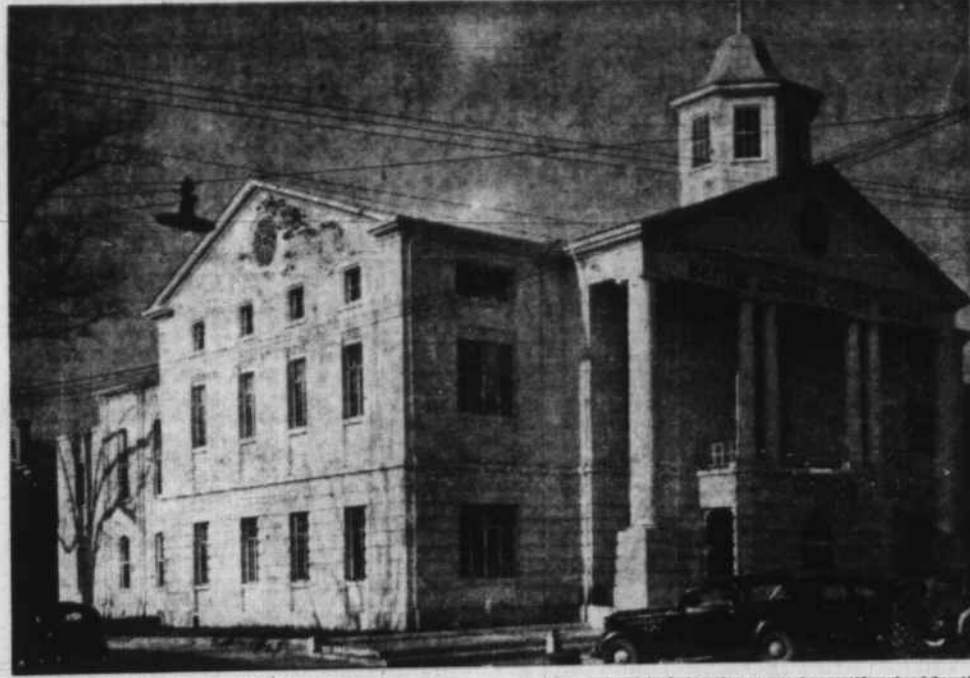
Bertie County has completed the transformation of its courthouse at Windsor. The court house had for a long time been inadequate in size and in bad repair. With the expenditure of $40,000 for materials and the wages of WPA workers, three wings have been added to the structure, the inside thoroughly renovated, and the exterior painted. The Bertie County commissioners sponsored the WPA project which has filled a long-lasting need in the county.
