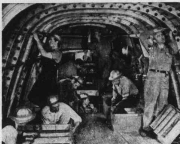
This looks like a vehicular tunnel, but actually it is the pilot's compartment of the 80-ton Douglas B-19 bomber, world's largest airplane, which is nearing completion in Santa Monica, Calif. The $2,000,000 craft will have the greatest load-carrying capacity, longest flight range and most powerful armament of any sky ship ever built.
