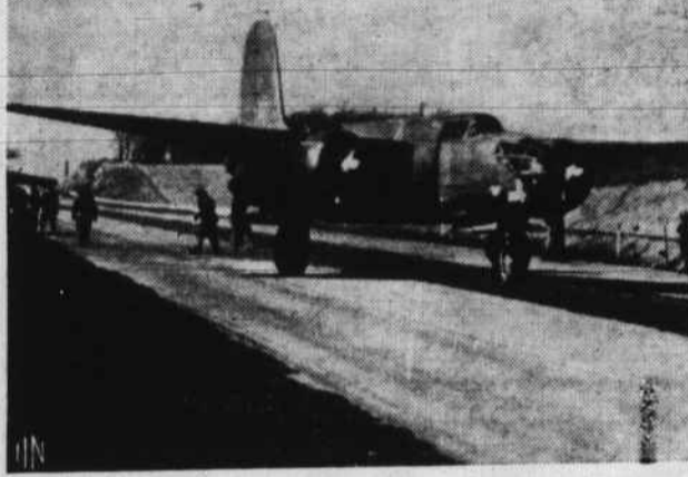
Motorists will have to keep their eyes on the sky as well as the road these days. The War Department has started on construction of flight strips which will be used as auxiliary landing fields. In the photo above an army plane straddles the dual Pennsylvania Turnpike after a forced landing. The flight strips would serve in such emergencies.
