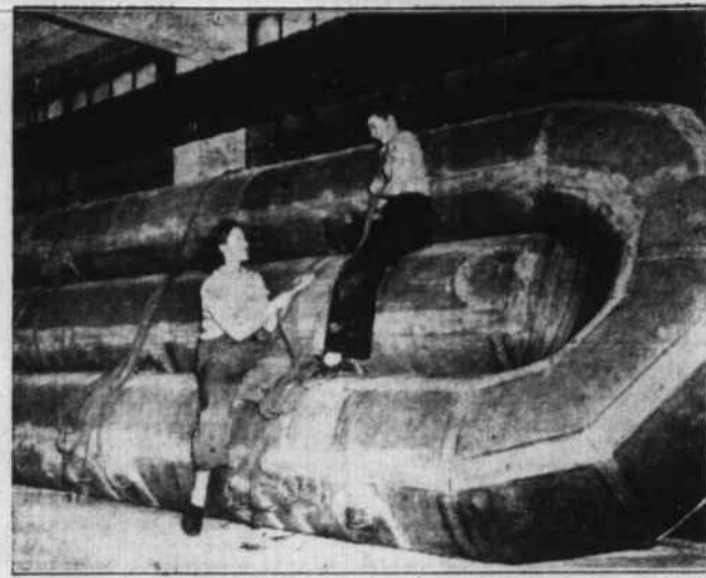
Massive rubberized cotton pontoons like the one above aid in giving added mobility and striking power to U. S. armored forces. By the use of such pontoons with heavy steel treadways, new armored force bridges can be erected faster and carry heavier loads than any other military bridge in existence.
