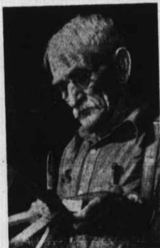
Seventy-one-year-old F. E. Lickey was 33 years old when the Wright brothers made their first successful flight, but he still isn't too old to be working on planes today. An expert woodworker, he's shown fixing a tail section of a cargo glider at the Boeing plant in Wichita, Kan. Five other members of his family also work at the same plant. (Central Press)
