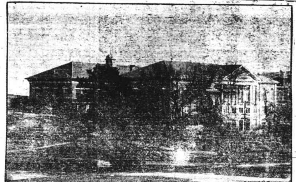
More than 1600 students can be fed at one time in this spacious dining hall at North Carolina State College. The additional wing, recently completed, is an exact duplicate of the old building, and it is erected immediately to the rear. The two units are connected by large serving pantries extending along each side of the central kitchen. The building, which is modern in every respect, including its own bakery and refrigerating plant, will be used for the first time at the opening of college, Sept. 4th.
