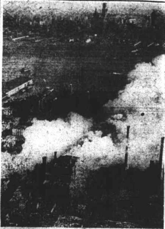
This is a remarkable airplane view of the $5,000,000 Jersey City, N. J. fire, at its height. More than 1600 families were made homeless. It is estimated, when a dozen tenement houses were destroyed. Three larger structures also were razed. Firemen from Jersey City, Hoboken and Newark fought the flames for several hours before the conflagration finally was brought under control.
