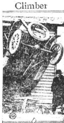
Climber After climbing an embankment six feet high and running 15 feet across the lawn this "Climber" made a desperate effort to climb on over a house at Vincennes, Ind. The car was stopped with its front wheels in the air and the driver intoxicated. was taken to the state farm to sober up.
