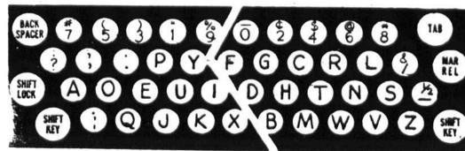
A NEW ARRANGEMENT of the typewriter keyboard (shown above) designed by Lt. Comdr. August Dvorak, Navy motion study expert, increases a typist's speed by approximately 35 percent. The line has been drawn to show the keys to be fingered by the left and right hands.
