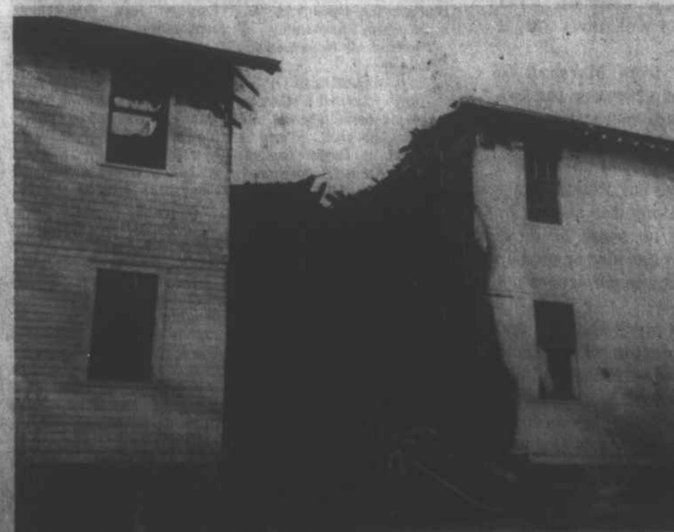
TREAT HALL, the 71-year-old dormitory on the Mars Hill College campus, was gutted by fire early Wednesday morning of last week. No students were residing in the wooden structure
