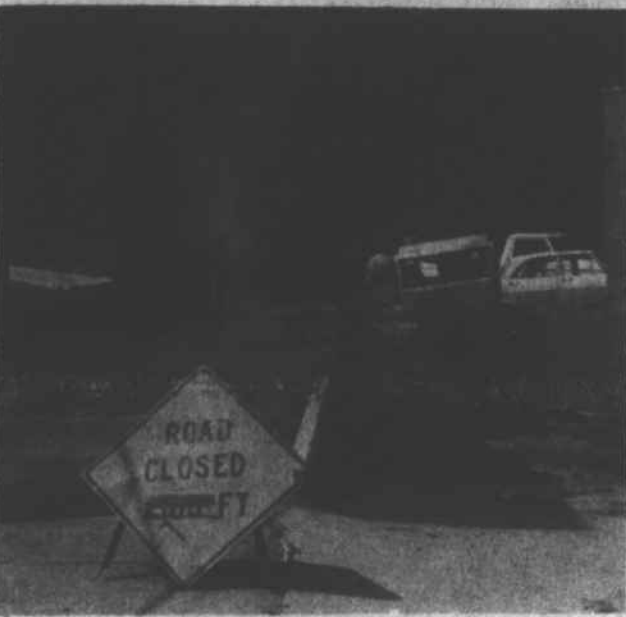
WORK ON THE SEWER PROJECT began on Hill Street Monday afternoon.
