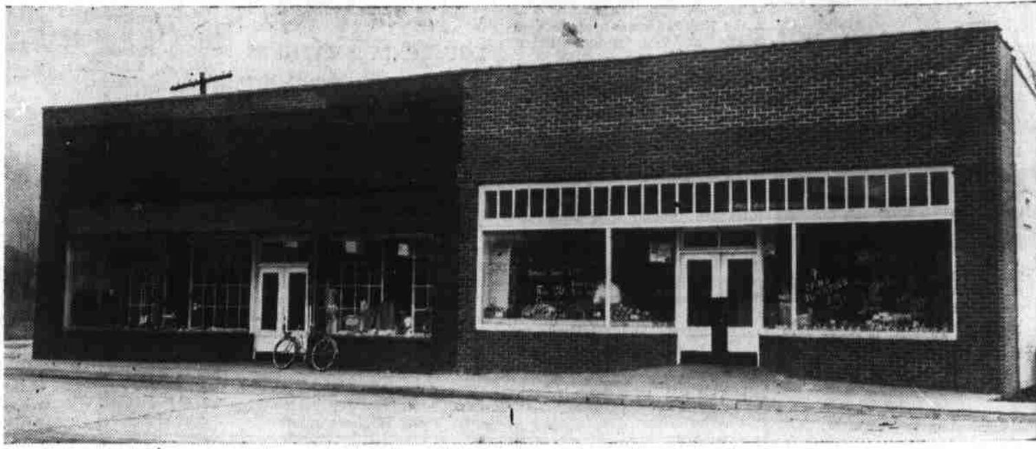
The firm of E. H. Balentine & Co. has about 6,000 square feet of floor space. Above is the general store, with the grocery and meat departments on the right, and the shoes, dry goods, clothing and notions on the left side of the building. The paint and hardware departments are in the rear. Furniture is carried in a separate building across the street, where ample display room is available. The feed and fertilizers are also housed across the street from the main store. The 12 departments carried by the firm are: clothing, dry goods, shoes, notions, ready-to-wear, hardware, paints, feeds, groceries, meats, fertilizers and feeds.
