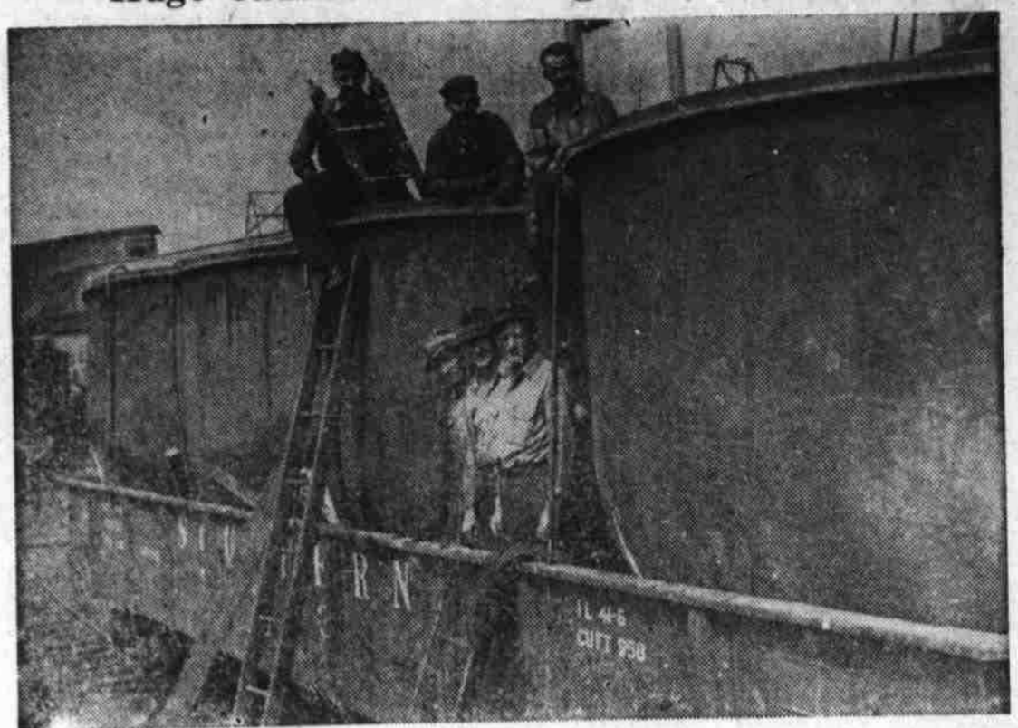
Shown above are four huge caustic pots averaging 14 tons each which were shipped as salvage by the Canton division of the Champion Paper and Fibre Company Monday morning. This is the second of two shipments totaling more than 100,000 pounds each made by the Canton plant in connection with the current scrap metal campaign. Members of the maintenance crew who assisted with the loading of the heavy pots are, from left to right: Top, Charlie Deaver, Rufus (Doc) Allison, and George Ingie; bottom, C. N. Carpenter, L. F. Pace, and F. F. Dotson, crew leader. (Photo by C. R. P. Cash.)
