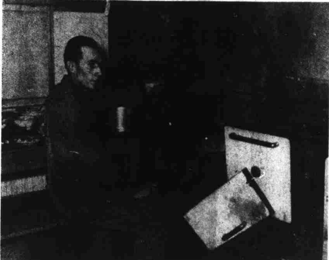
Results of the explosion, on the morning of February 5th, of the water tank behind the kitchen stove in Ben Medford's home are apparent in the picture above. Mr. Medford is shown pointing to a large hole in the side of the house (some boards were laid over it when the picture was taken). He and seven other members of his family were sitting at the table eating breakfast when the tank blew up, but no one received serious injury.—This is a Mountaineer photo by Worthington, Skyland Studio.
