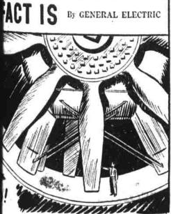
HURRICANE IS CREATED IN THIS WIND OFFETT FIELD, CAL. IT TAKES GENERAL NOTORS TOTALLING 27,000 HORSEPOWER BLADES SHOWN IN THIS PICTURE.
