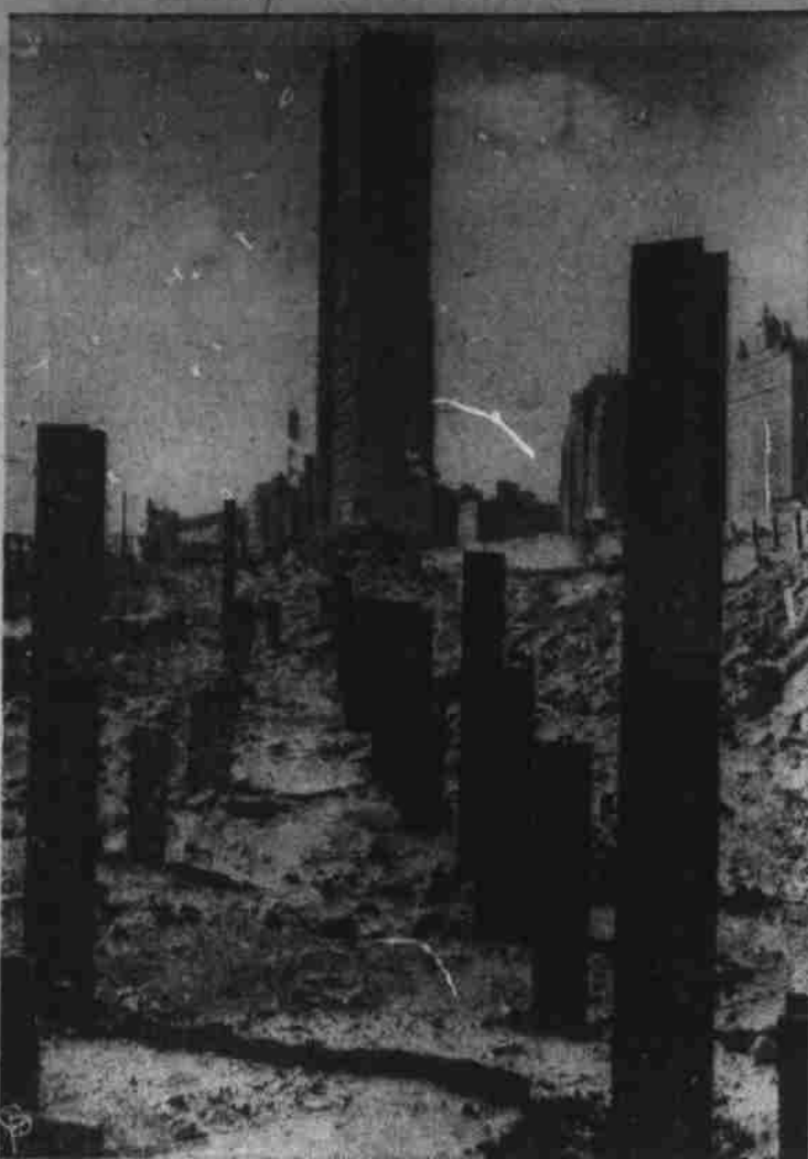
RISING IN STately ELEGANCE, the new United Nations Secretariat Building in New York is almost ready for occupancy. In the foreground of this future monument to world peace are rows of steel posts marking the sites of other U.N. structures which will soon be erected. (International)
