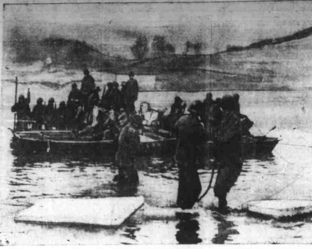
KEEPING CLOSE ON THE HEELS of hard-pressed Chinese Communist and North Korean troops, members of the Third Combat Engineer Battalion are carried across the icy Han River on a ferry constructed of four boats. The river has been bridged in several places by U.N. troops as they extended beachheads. (International)
