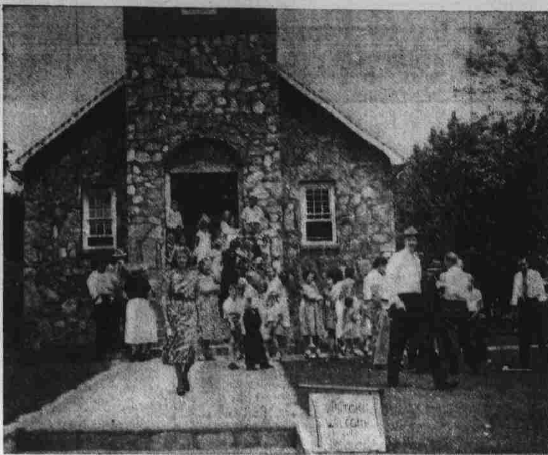
This is the new rock building of the Green Valley church which burned the last note on the building the 19th. The church was organized in July 1949. Has 125 members, and 143 in Sunday School, with George Troutman, superintendent. (Joe Davis Photo).
