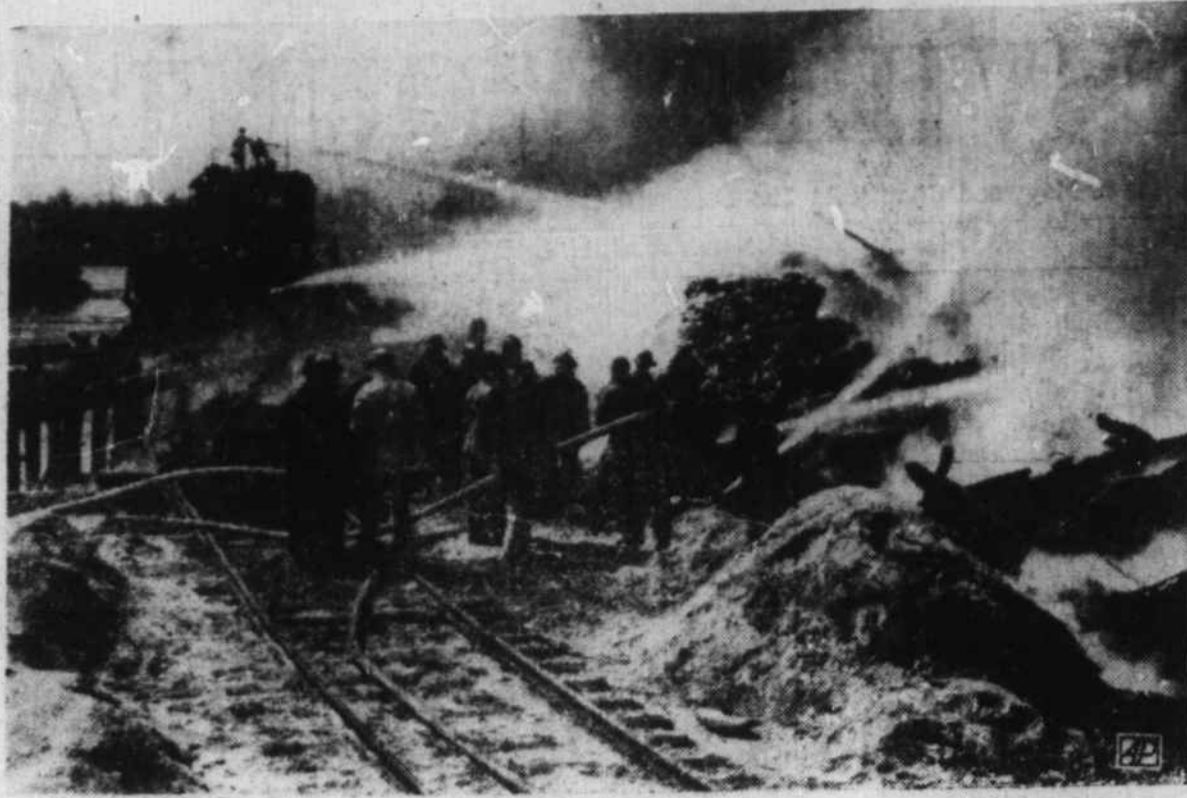
Firemen pour tons of water into the smoldering ruins of a quarter-mile stretch of waterfront at Wilmington, where a wind-swept blaze caused damage estimated as high as 30 million dollars. A fire-boat at left joins in the fight. Twenty-one persons were treated at hospitals as a result of burns and injuries caused by the fire. (AP Wirephoto).
