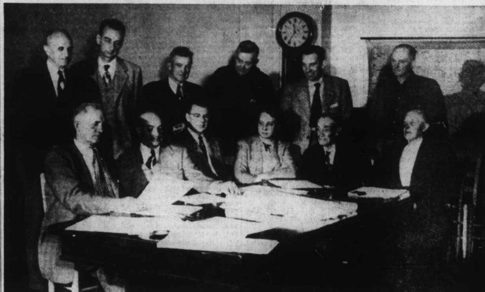
Last Friday county officials formally awarded contracts to low bidders for construction of the Central Elementary School. Seated from left are C. C. Francis, chairman of the County Board of Commissioners; W. R. Francis, county attorney; Jack Baber of Asheville, architect in charge representing Lindsey Gudger; Mrs. Lucy Jones Boyd, superintendent of county schools; J. W. Killian, chairman of the Board of Education; and Jarvis Allison, county commissioner. Back row: Letch Worley, member of the Board of Education; J. R. Sechrest of Canton, member of the Advisory Board; Frank M. Davis, county commissioner; Gwyn Denton, architect; Dave Felmet, chairman of the Advisory Board; and Glenn Brown, member of the Advisory Board. (Mountaineer Photo)
