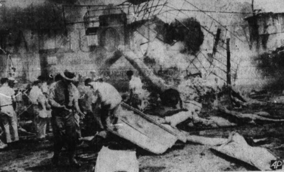
OIL PLANT EXPLOSION KILLS 1, INJURES 3 —Rescue workers search the wreckage of the High-Penn Oil Co. refinery near Greensboro, for the body of Rufus Whitaker of nearby High Point who was killed in an explosion. Three other men were injured by the terrific blast and fire which destroyed the plant. Whitaker's body was found later under tons of debris. The cause of the explosion was a mystery. (AP Wirephoto).
