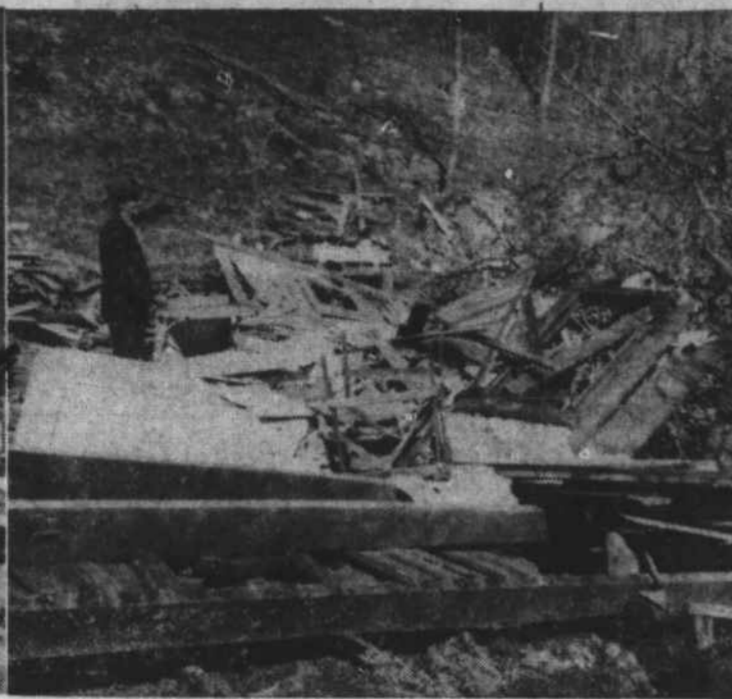
HEAVY OBJECTS such as an electrical refrigerator (foreground) and a cook stove (not shown) were thrown together in a heap by the force of the twister which destroyed five buildings owned by Alfred Johnson on McClure Creek in Cecil community. At right are branches of a tree uprooted by the house as it was torn from its foundation. (Mountaineer Photo).
