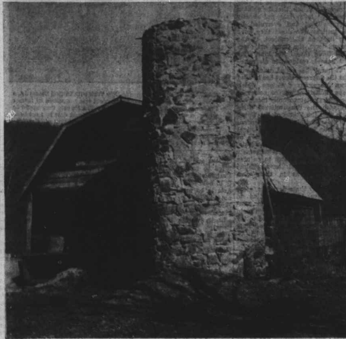
ONE OF THE FEW natural-rock silos in Haywood County is this one on the farm of J. Edgar Burnette of Cecil Community, situated near the intersection of the Lake Logan and McClure
