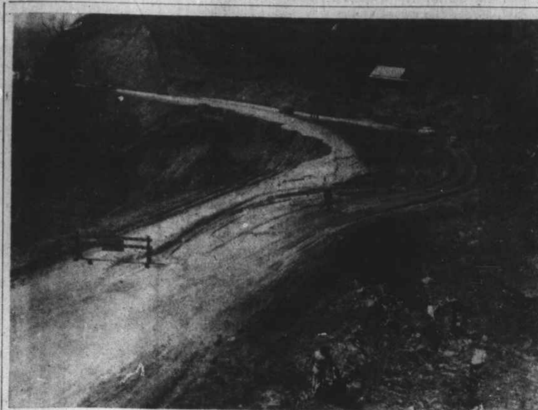
ABOUT 50,000 cubic yards of earth comprising the "toe" of a large fill on US 23-441 between Franklin and Sylva gave way about 3:30 Monday afternoon. The tons of earth slid down to the valley below. The slide occurred about seven miles from Franklin, just below Cowee Gap at the Macon-Jackson line. A bulldozer cut a temporary by-pass around the danger zone. (Photo by Sylva Herald).
