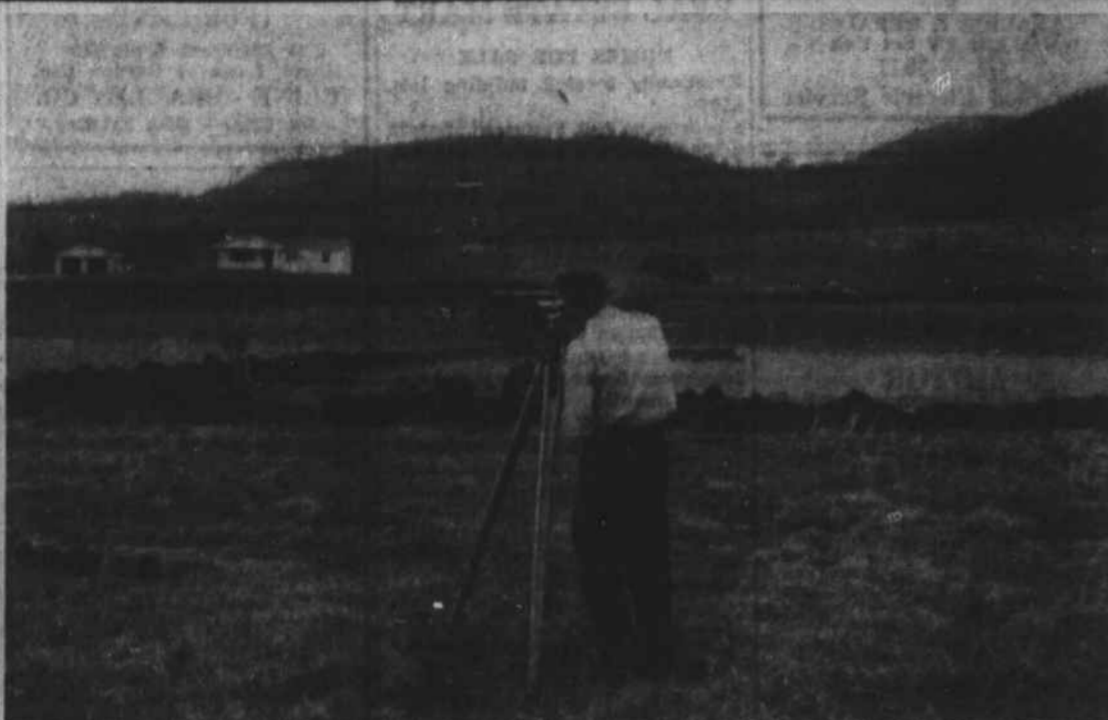
ROY BECK, work unit soil conservationist in Haywood County, is shown here making a survey in connection with the installation field drain tile on the farm of Ray Davis in Beaverdam Community. In the background holding a sighting rod is Carlisle Davis, conservation aide. (Soil Conservation Service Photo).
