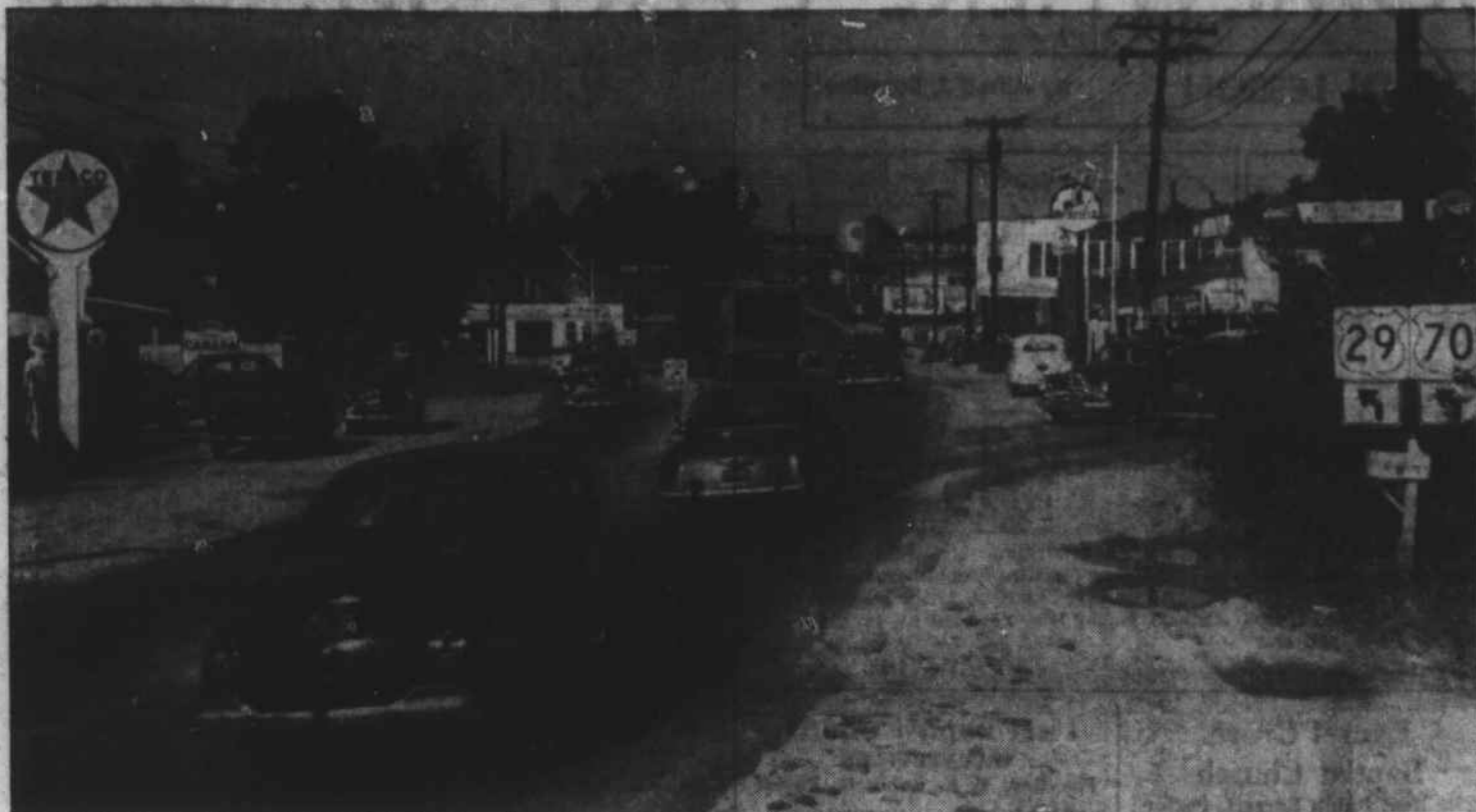
CONFUSION AT THE CROSSROADS —This congestion is being relieved in North Carolina communities by the construction of limited access highways which provide for the free flow of traffic without the penalties of uncontrolled entrance and exits. The
