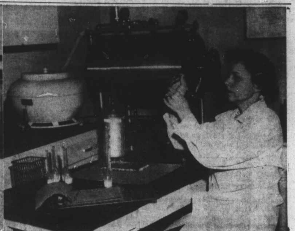
BUTTERFAT CONTENT of retail milk samples is estimated by the Babcock test, being made here by Mrs. Rebekah Murray, bacteriologist at the Haywood County Health Center. This is one of a number of safeguards maintained by dairies and the Health Department to insure the purity of milk sold in the county.
