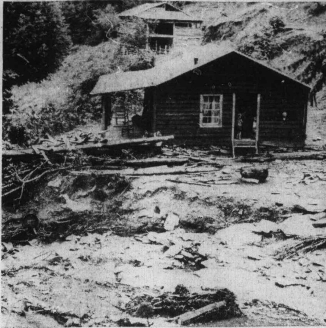
GRIM REMINDERS of the flash flood at Cove Creek are these logs (left) and rocks left in the yard of the home of Mr. and Mrs. Lloyd Sutton, situated only a few yards from the creek which overflowed its banks. Had the foundation of this house been less sturdy, the entire structure probably would have swept away by the swift flood waters.
