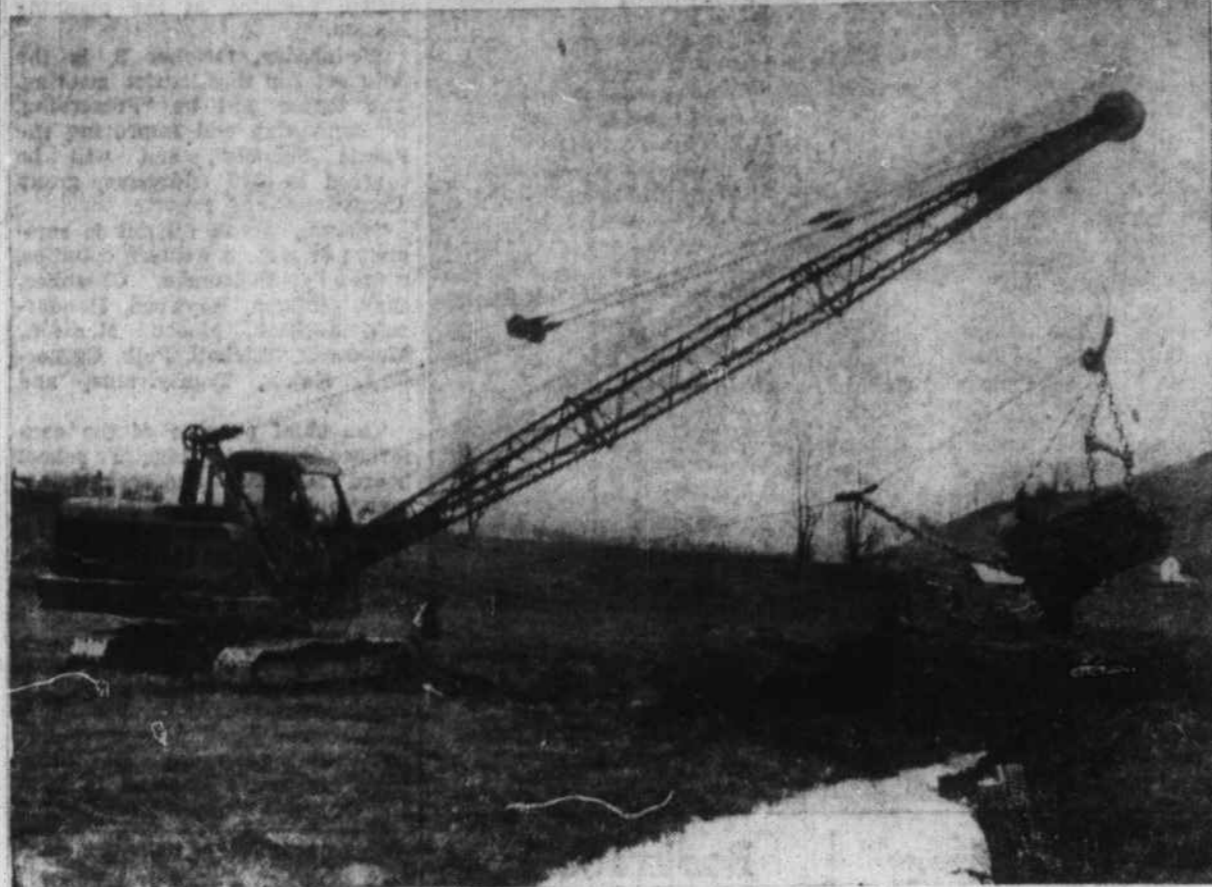
OF SPECIAL INTEREST in Haywood County at present is the widening and deepening of creeks to provide faster runoff of water to avoid flooding during heavy rains. Such a project is now planned in the Cove Creek area. This picture
