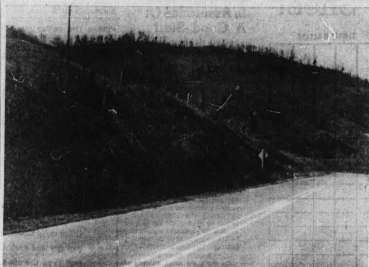
KUDZU GRASS has been used to halt erosion on this roadbank along the Crabtree road near the residence of Albert McCracken. Seeding of roadbanks is one of the major projects being
