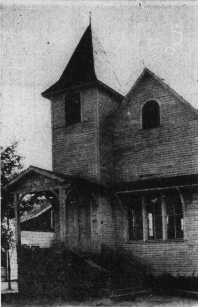
THE HAZELWOOD METHODIST CHURCH, established as a mission about 15 years ago, has outgrown its quarters. Members are setting aside funds for a new building. (Photo by Elliot Lyman Fisher).
