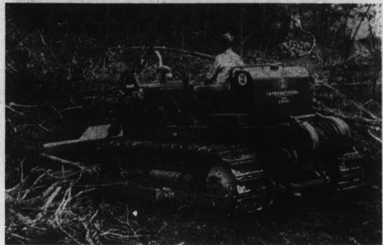
MODERN METHOD of clearing farm land is by bulldozer, such as this one owned by Joe Palmer and operated by Ed West. Under contract to Frank Davis, Iron Duff dairy farmer, the bulldozer cleared some 10 acres of land in 25 hours—a job
