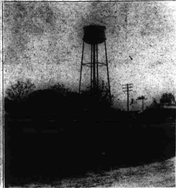
The above is a scene of the new water tank recently erected to serve the citizens of Faison. Water and sewage has long been a great need of this town and after years of dreaming it has become a reality. The tank is located just back of the Faison Garage.
