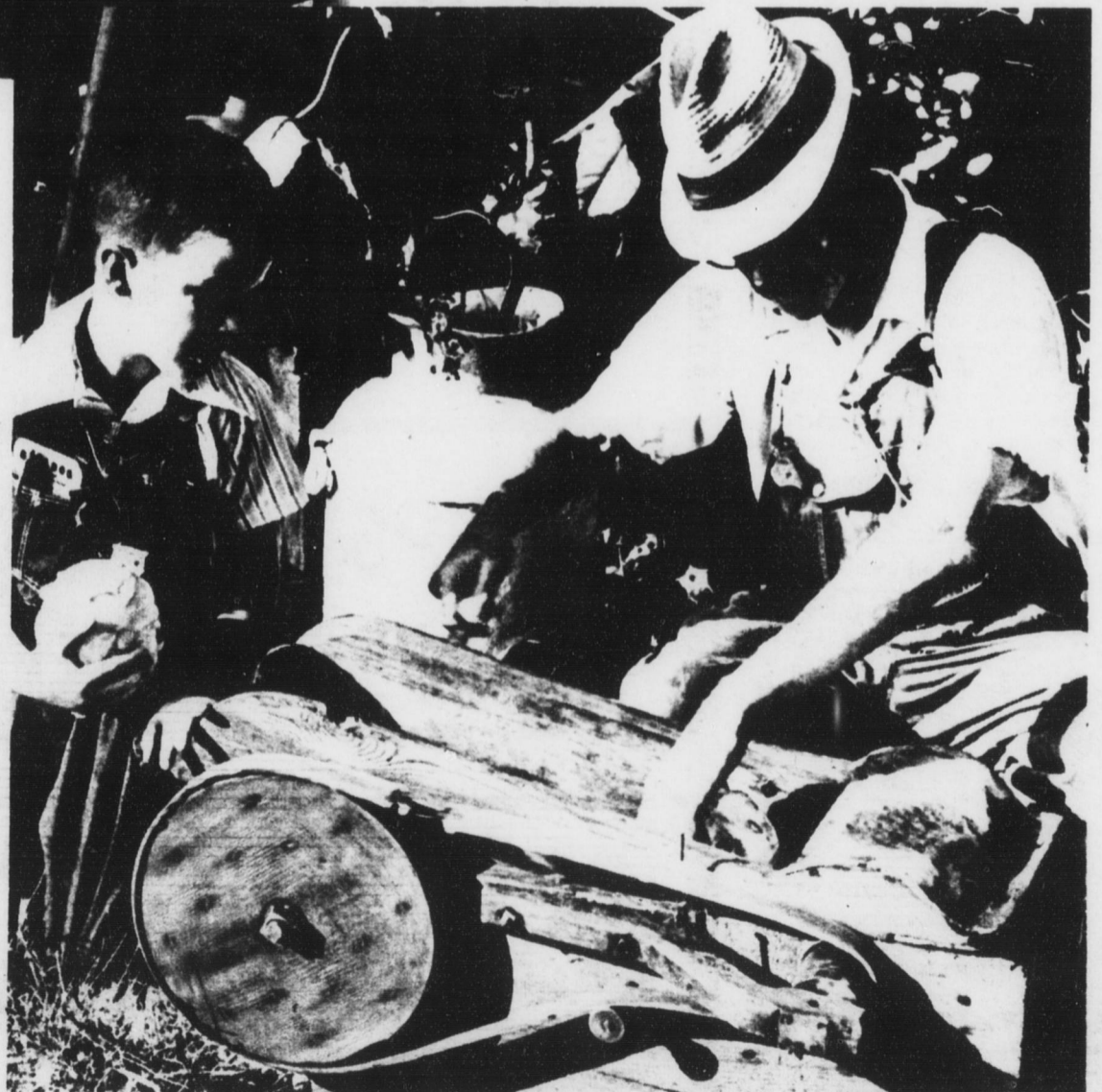
CABBAGE CUTTER — Roy Nolley and his grandson Mark Hancock feed cabbage into a cabbage cutter. The unusual old machine is used for making cabbage into sour kraut. (Staff photo by Barringer).
