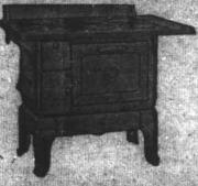
Large Range, Six Caps, Semi-enamel, made of finest grade Southern east iron, durable flue-con-struction, oven thermometer, large fire box with heavy liners and duplex grates.
