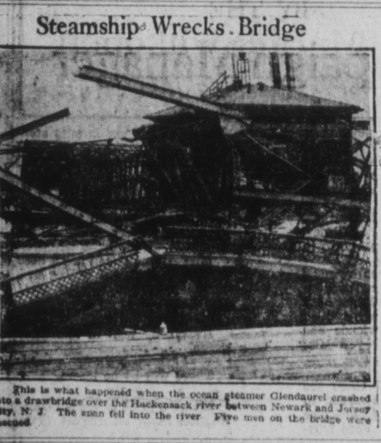
This is what happened when the ocean steamer Glendaurel crashed into a drawbridge over the Hackensack river between Newark and Jersey City, N. J. The men fell into the river. Five men on the bridge were rescued.
