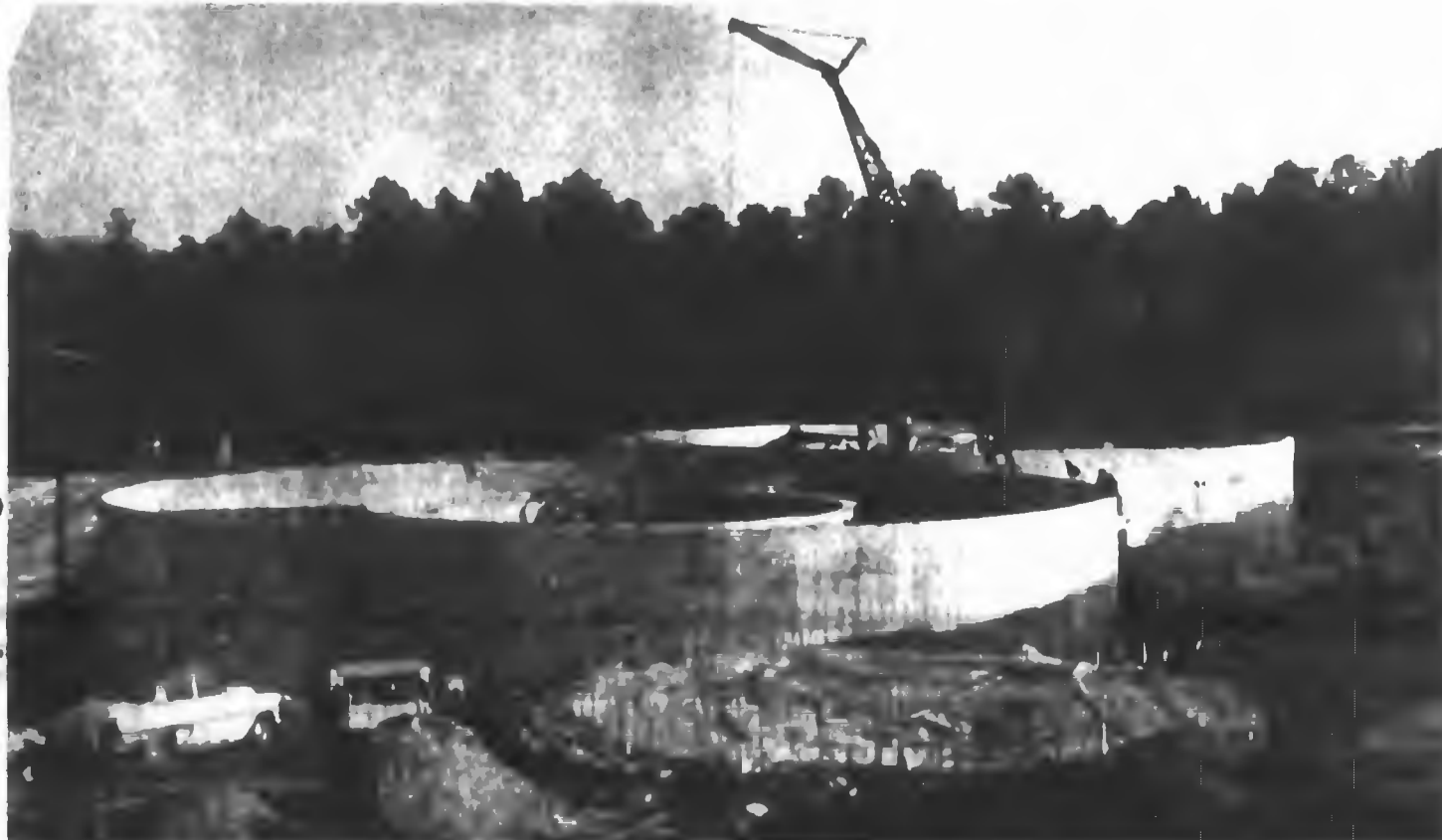
New Town Sewage Disposal Plant
