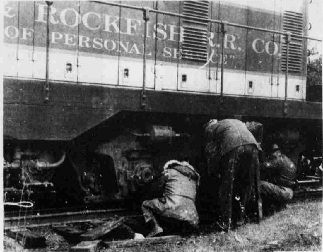
TRACK JUMPER - An Aberdeen and Rockfish railroad car attracted considerable attention Tuesday when it jumped the track at the Elwood Avenue crossing (apparently for no reason at all). Sidewalk overseers contributed a lot of peering and pondering over the situation but believe it or not, the heavy iron wheels were guided by three railroad workers from their position between switch tracks onto the rail with wooden boards and scantling.
